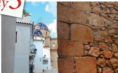
Remains of la muralla del Baluarte
