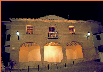
The Main Hall in the Teulada Law Courts
